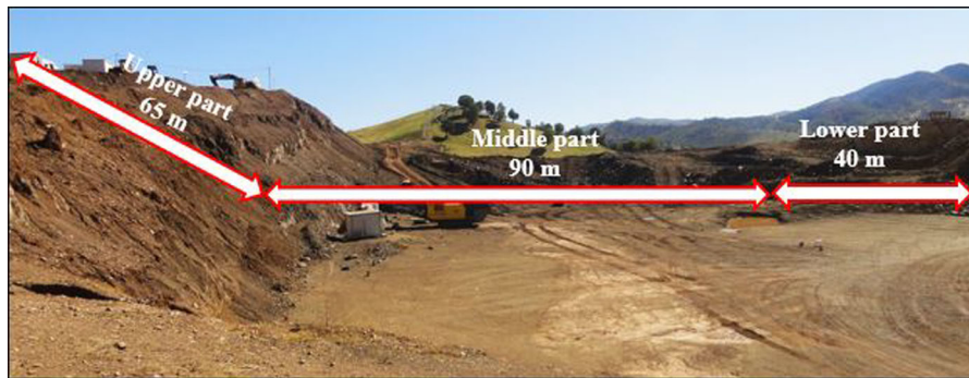
Fig. 2 General view of the Sharbazhar Quarry looking north eastwards and showing three parts
