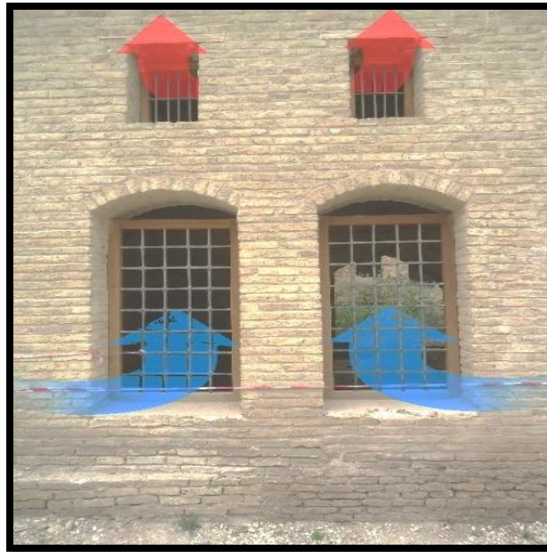
Figure 6: Windows ventilation mechanism
