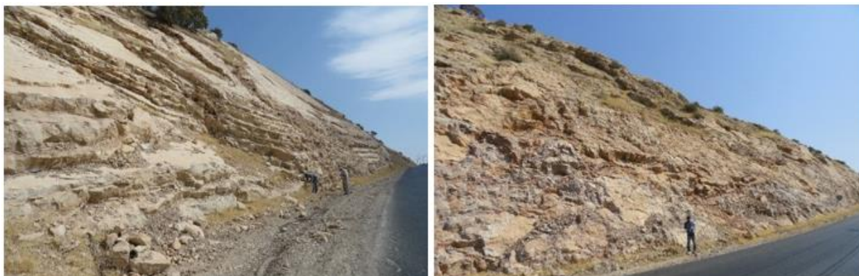
Fig. 4. Road Cuts with well bedded, carbonate rocks of the Pila Spi Formation where bedding planes daylight in the slope face (Station No. 7)
