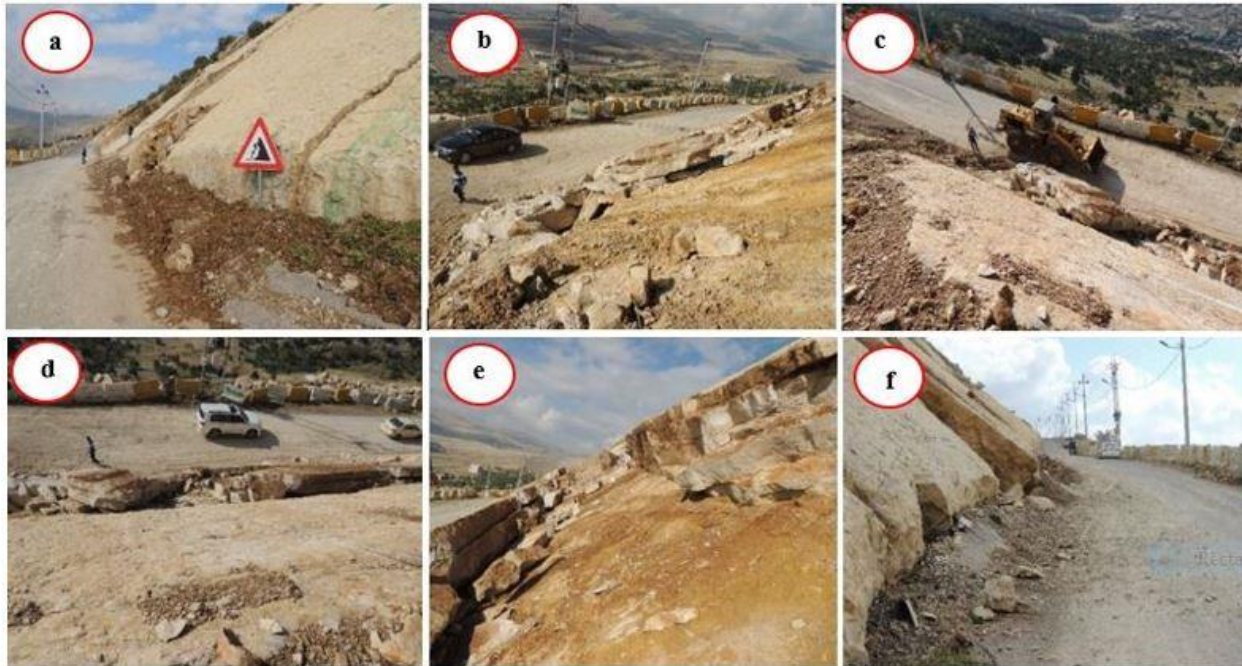
Fig. 3. Landslide of 11 November 2015 at Haibat Sultan Mountain. 3a) Traffic sign for rock falls indicating continuous landsliding, 3b) Large slid blocks, 3c) Top view of the landslide, 3d) Top view of the landslide, note the damaged road fence; in the back ground, 3e) The shear plane of sliding, 3f) Toe of the landslide, note the road had functioned as a retaining wall to stop the sliding of the rock blocks.
