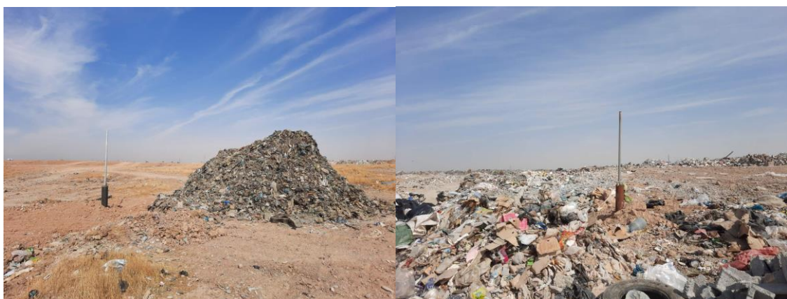
Figure 7: Gas collection pipe at ELS (Visited on 28 October 2020)
