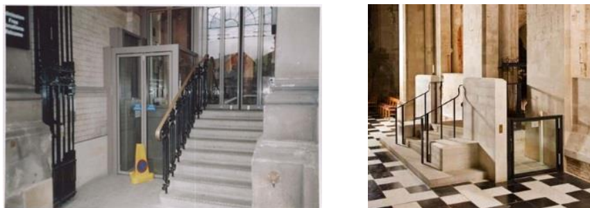
Figure 5: (a) Vertical platform lift at the Grosvenor Museum, Chester [23], (b) Vertical platform lift at Albans Cathedral [21].
