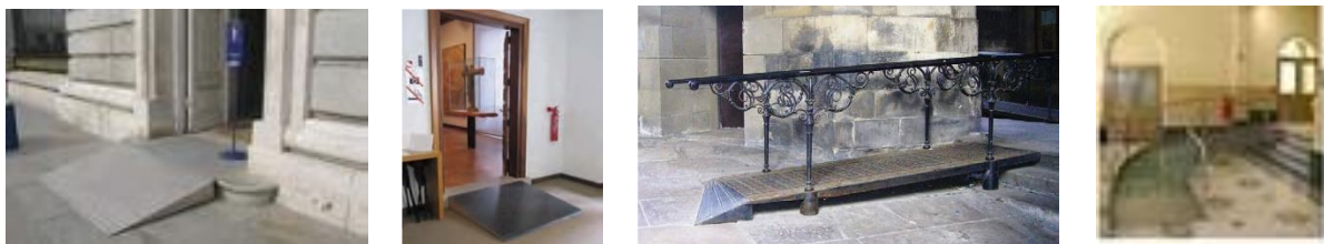
Figure 1: Ramps (a) Exterior portable [14], (b) Interior portable [16], and (c) Exterior semi-permanent [17], (d) Interior semi-permanent [18]
