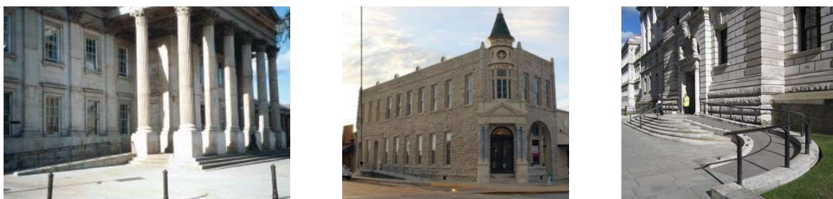
Figure 2: Permanent entrance ramp (a) Straight ramp [19], (b) Straight ramp to new entrance [20], (c) Curved ramp [21].
