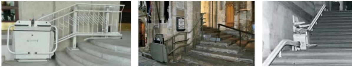
Figure 6: Inclined lifts (a) Exterior stair climber lift [21], (b) Interior stair climber lift [16], (c) Interior chair lift [19]
