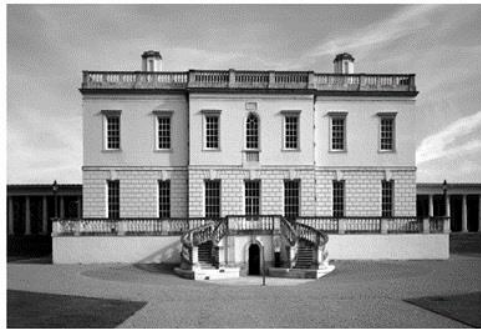
Figure 3: Queen's House, Greenwich; the access solution is by creating a level entry into the basement via an existing door opening [22]
