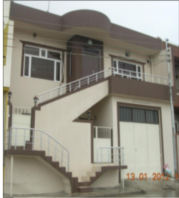
B: Front view of the house
