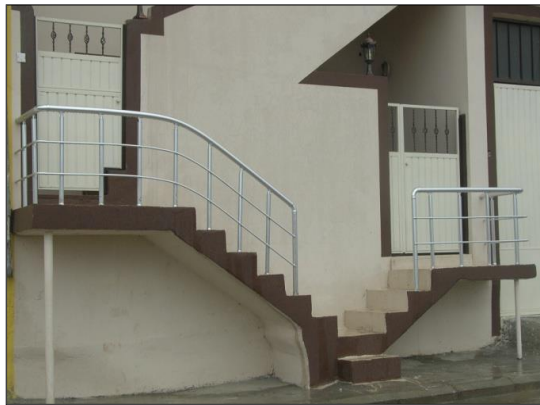
D: View of the two external stairs with a common space between them where the space is 50cm and taking the outdoor walk way (Prepared: Researcher)
