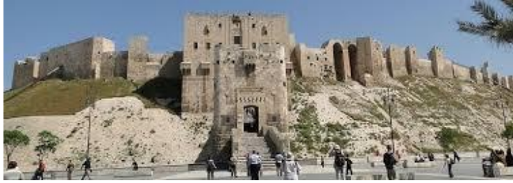
FIGURE 1. Slope and Stone Cladding Ref.: Internet
